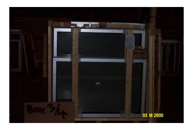
2.6 Lift the window by putting a suction cup on the exterior light of glass. This will be marked.
