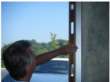
2.15 Plumb the four sides of the window in the opening using a level. Use plastic shims between the frame and the wall.
