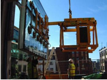
2.9 now place suction cup lifting device on the exterior glass and Transport the window to its installation opening. The window will be easily set by crane from the exterior of the building. If glass is the on the interior side you may lift from the interior side as an option. Do not place suction cups on polycarbonate.
